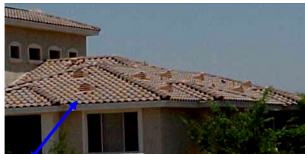
Dormer vents installed on a tile roof.
