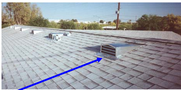
Dormer vents installed on a composite roof.
