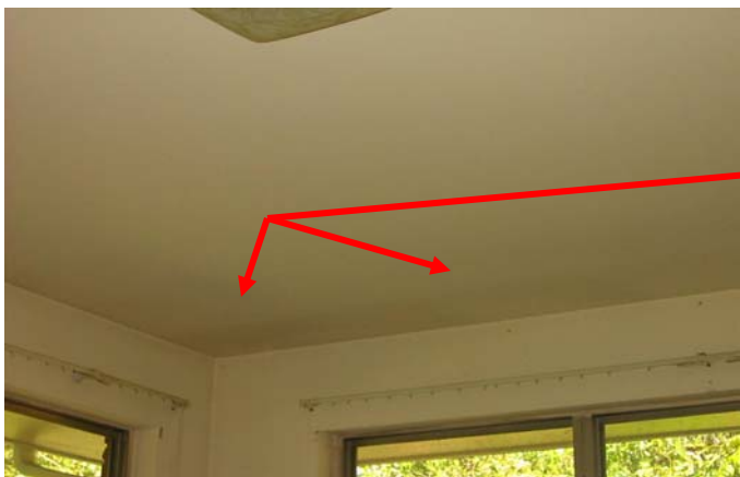
Master bedroom northeast corner ceiling.
